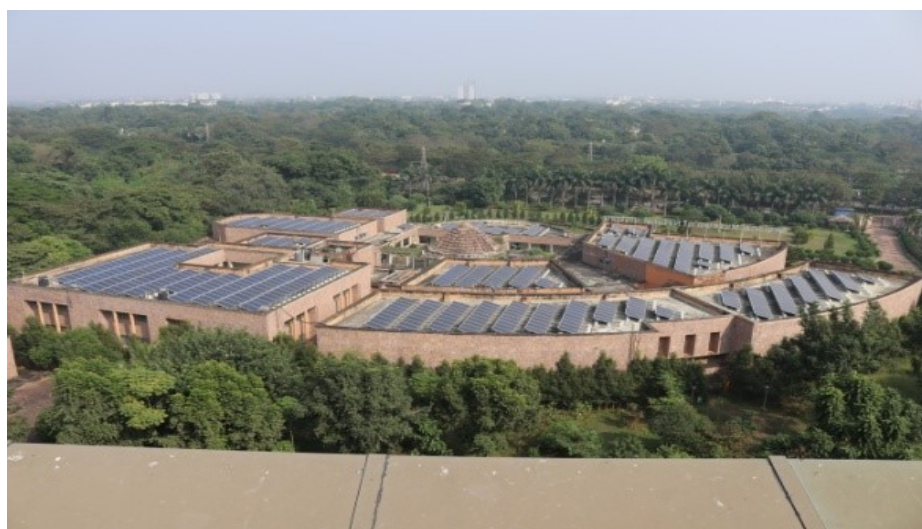
Figure-5 Roof Top Solar Power Plant, RMNH Bhubaneswar
